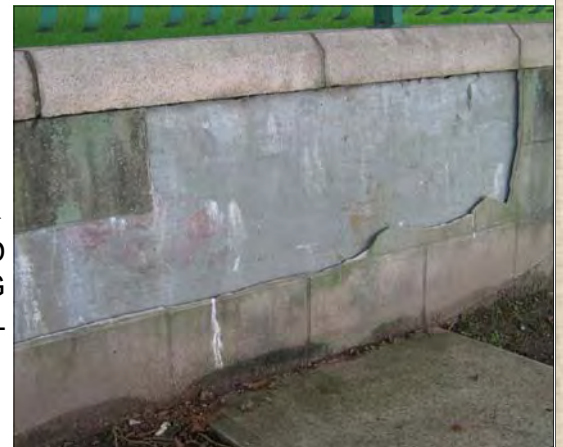
▶ EXPOSED RETAINING WALL
